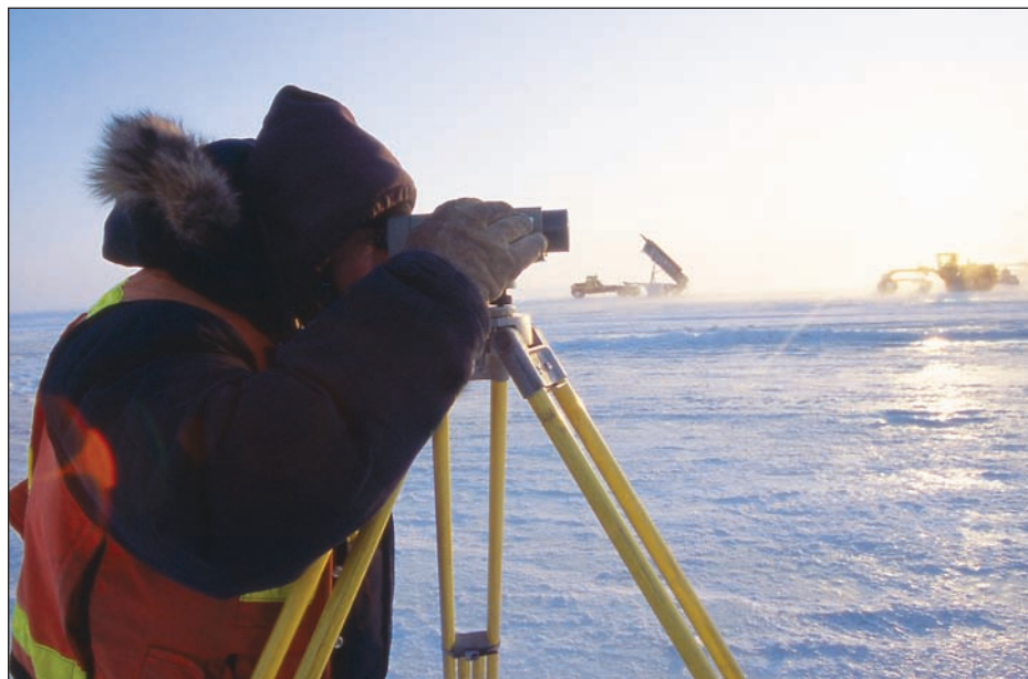
Lounsbury surveyor setting grades for ice pad construction
